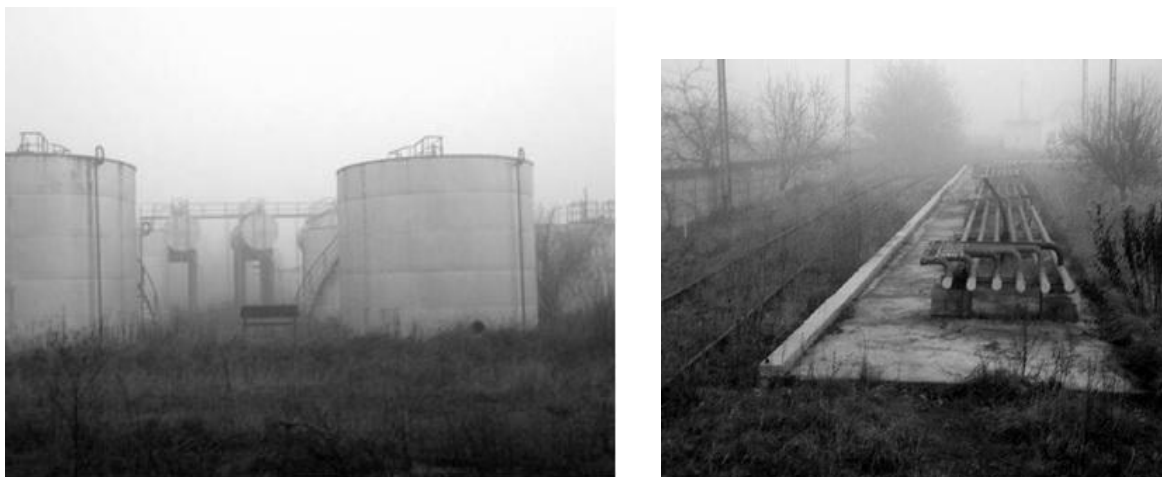
Figure 3 Deposit's condition before demolishing
